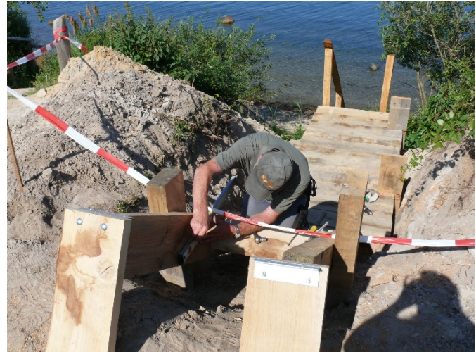
12 - tourism infrastructure construction – © BRASOR
