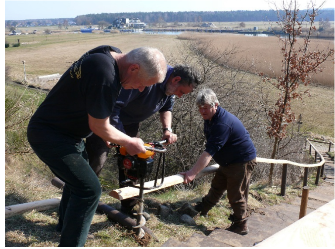
10 - Infrastructure maintenance – © BRASOR
