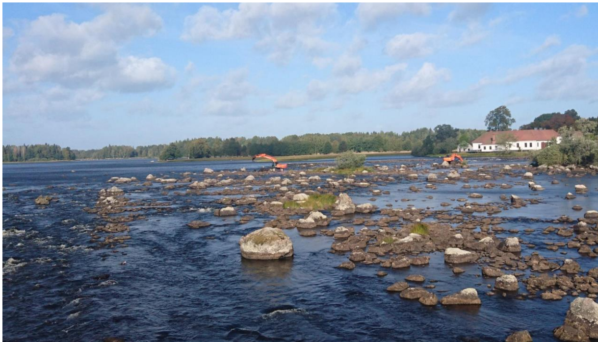
Two excavators restore the rapids at Gysinge.
