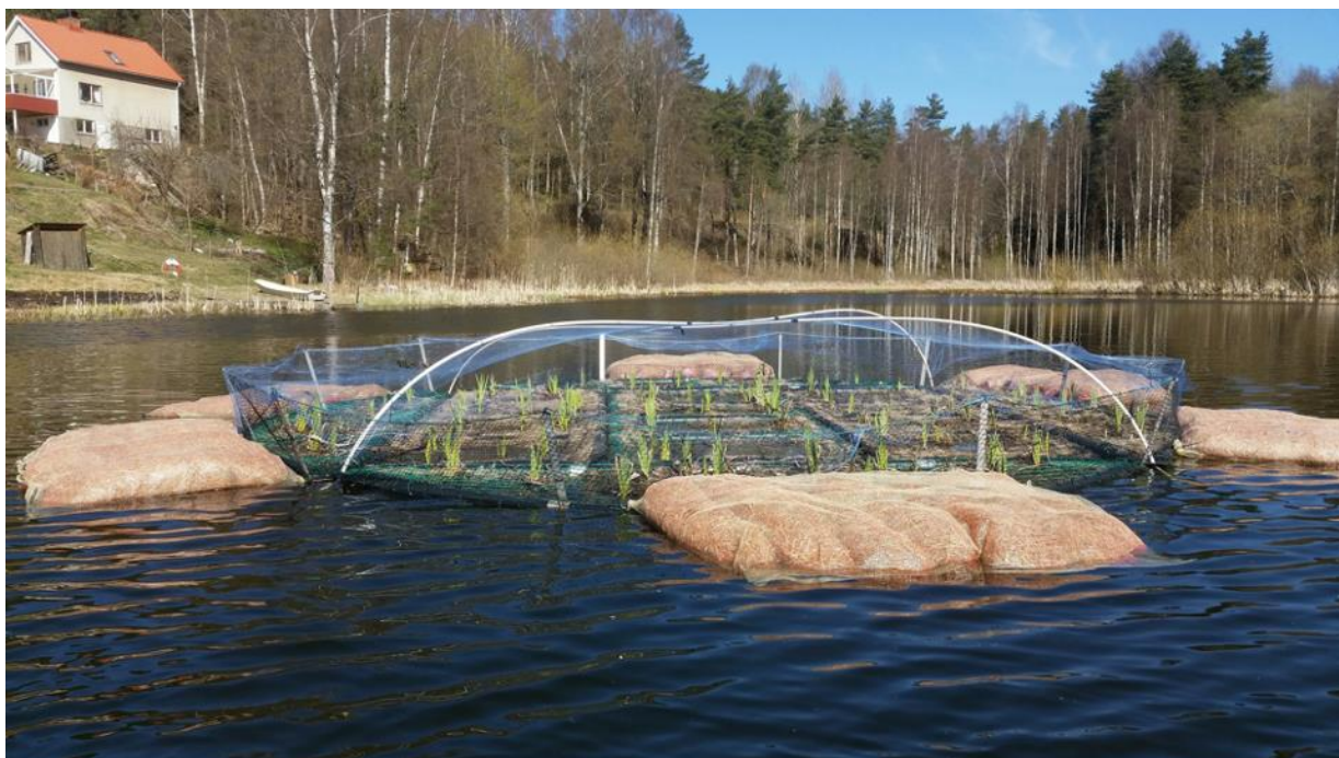
Floating islands used to purify the water in lakes.
